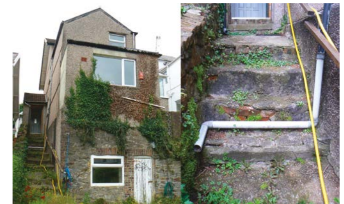
An example of poor housing issues addressed – this home has rear garden and garage access via steep steps that are in disrepair, slippery, and have rain water drainage discharging onto them.
